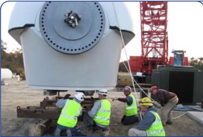
*Preparation of nacelle (generator) prior to placement on top of the tower.*
