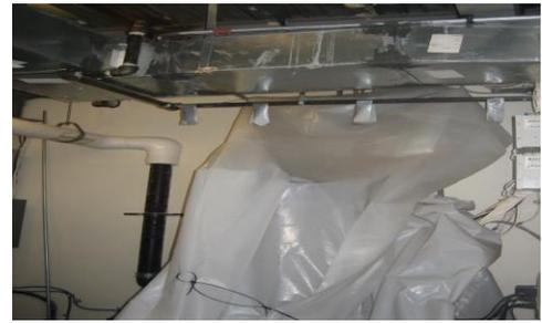
**3<sup>rd</sup> Floor Communications Room Roof Leak**
